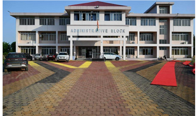
Administrative Block, Arunachal Pradesh University, Pasighat
